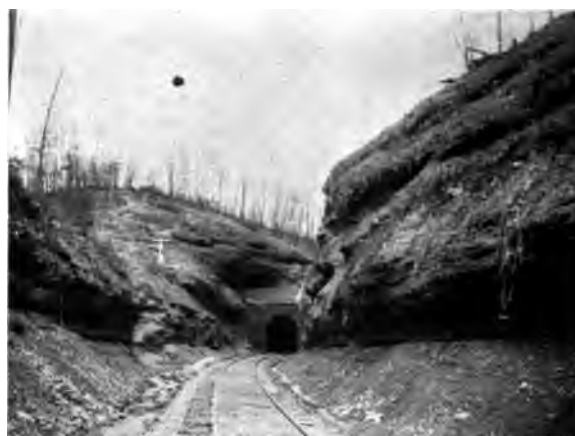
ENTRANCE TO KING'S MOUNTAIN TUNNEL.
